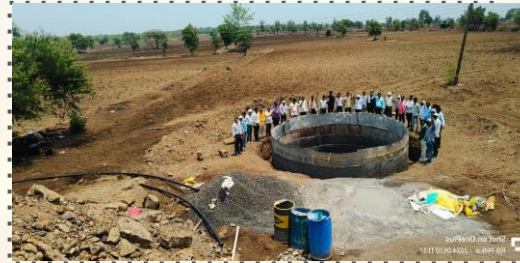
On field training about Well recharge through rainwater harvesting at Village Bhankheda
